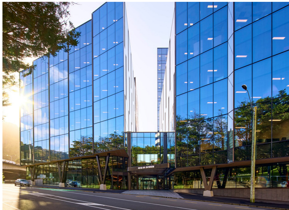
Bowen Street, Wellington 5-star Greenstar commercial building
